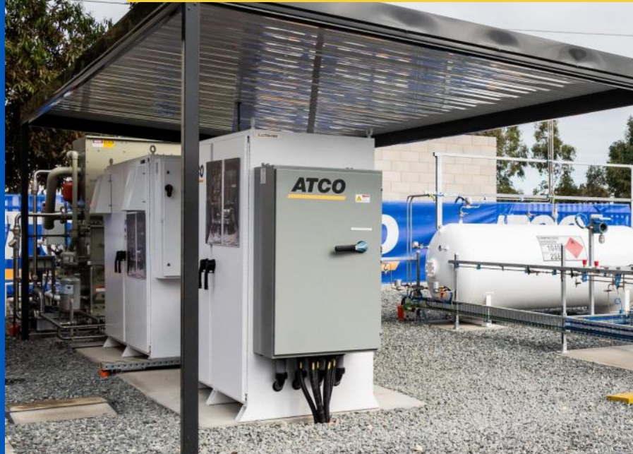
Clean Energy Innovation Hub - Western Australia
