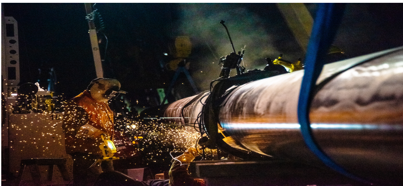
Pembina-Keephills transmission pipeline construction, near Wabamun Lake, Alberta
