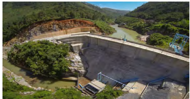
Hydroelectric power station, Veracruz, Mexico
