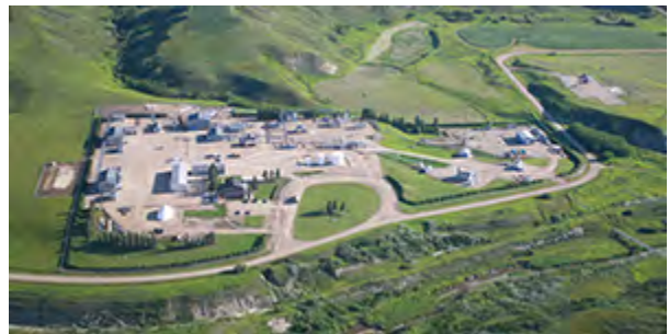
Natural gas storage facility, Carbon, Alberta
