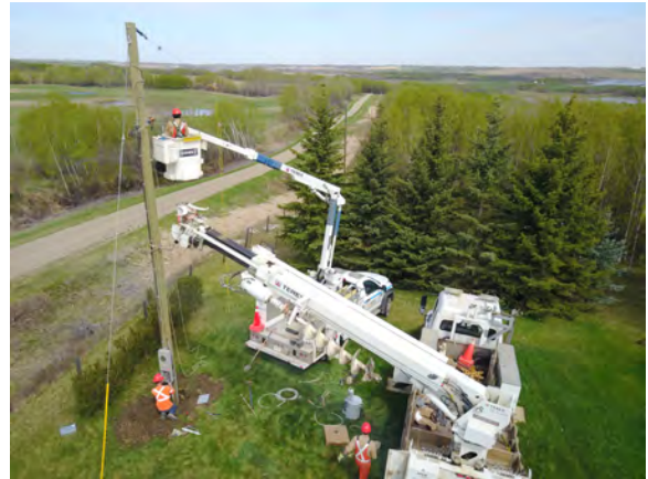
Electricity Distribution, Maintenance Work, Alberta
