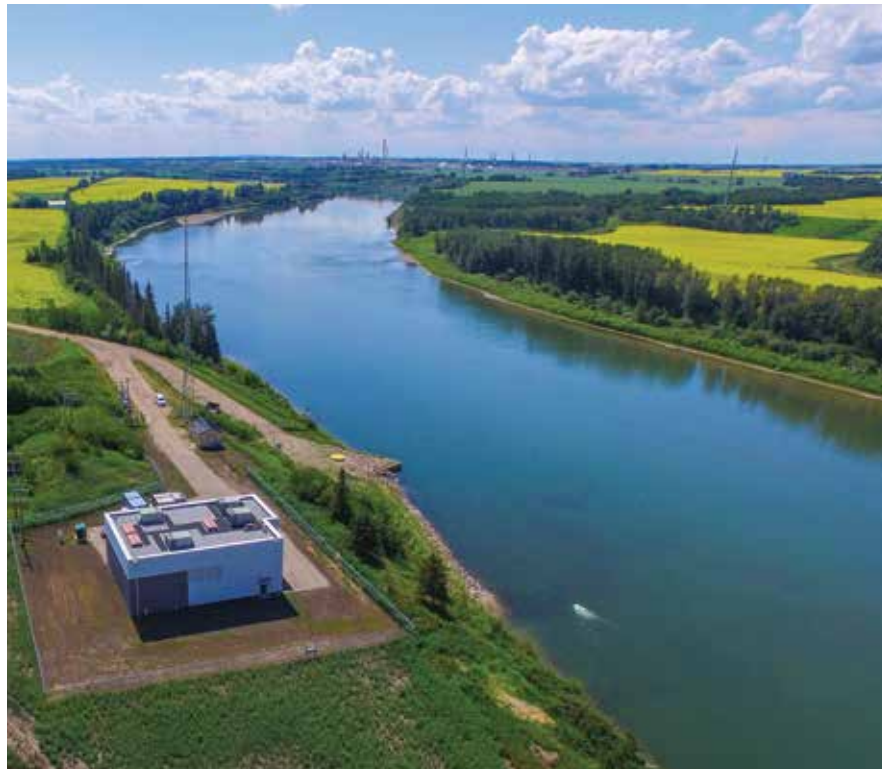
Over the last seven years, we have invested more than $70 million into projects that expand our industrial water system in Alberta's Industrial Heartland.
