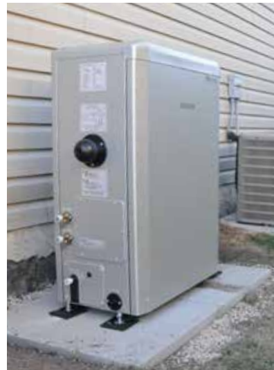
We are helping our customers reduce emissions and operating costs with Micro Combined Heat & Power technology, using onsite natural gas to efficiently generate heat and electricity. In 2016, we established a pilot program involving several Alberta homes and a natural gas regulating station to determine the viability of this new potential service offering.
