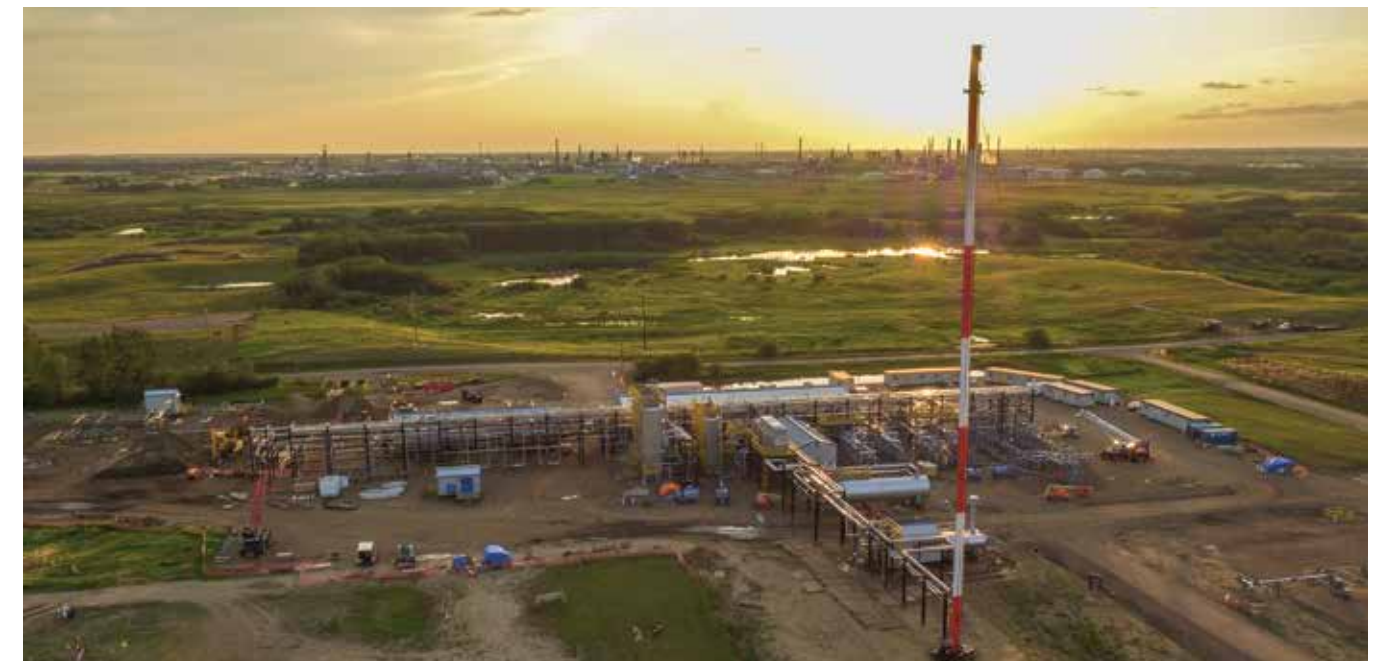
Our salt cavern facility at the ATCO Heartland Energy Centre allows us to leverage our industrial water infrastructure in the area to wash two caverns simultaneously which shortens development time. The central location also provides our customers with transportation options to solve the logistical challenges of moving product to market or securing it to avoid processing interruptions.
