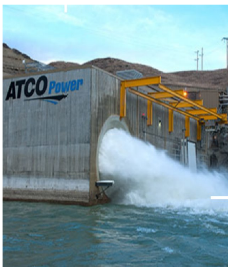
Oldman River Hydroelectric Plant
