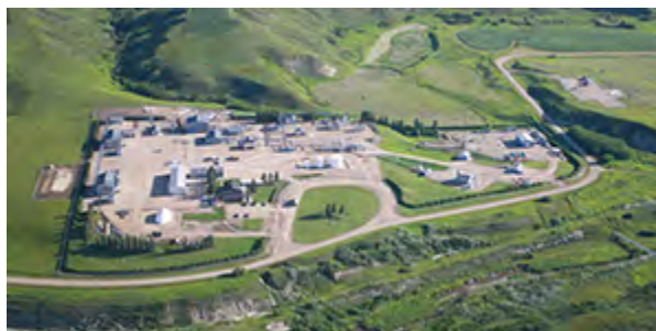
Natural gas storage facility, Carbon, Alberta
