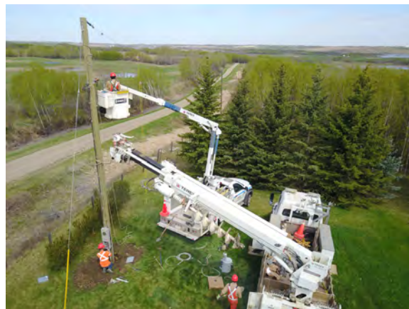
Electricity Distribution, Maintenance Work, Alberta
