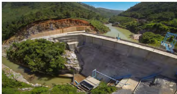
Hydroelectric power station, Veracruz, Mexico
