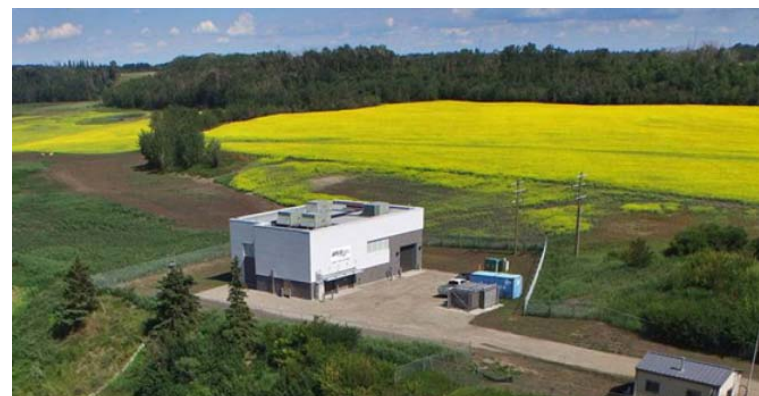
Heartland Industrial Water System
