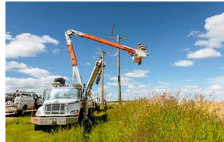
ELECTRIC DISTRIBUTION $2,476M Rate Base
