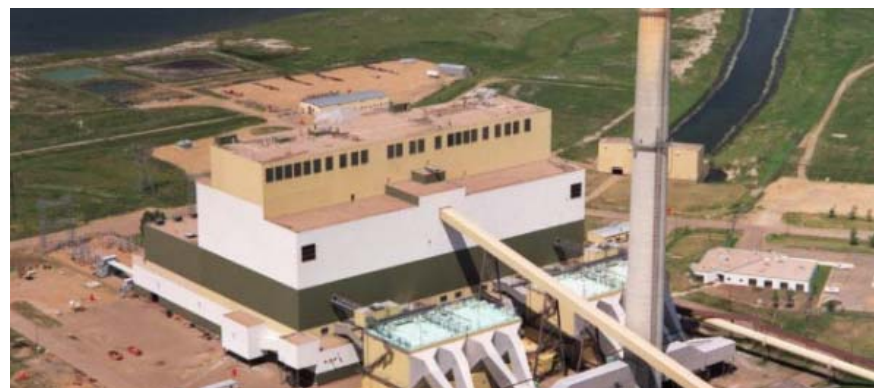
Sheerness Generating Station
