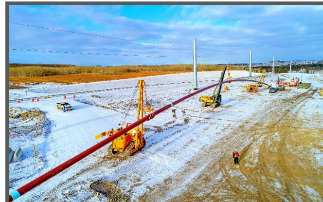
NATURAL GAS TRANSMISSION $297M
