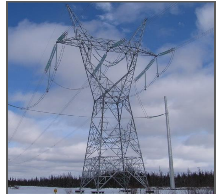
FORT MCMURRAY WEST 500 KV TRANSMISSION
